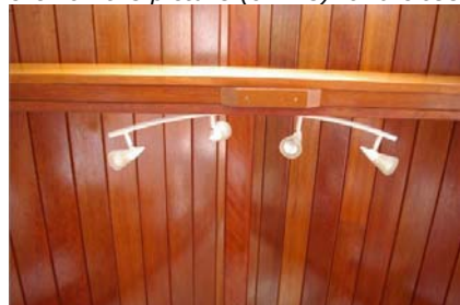
V" groove Sirari ceiling
