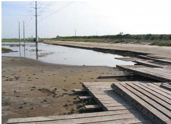
dragline and crane mats for heavy equipment support
